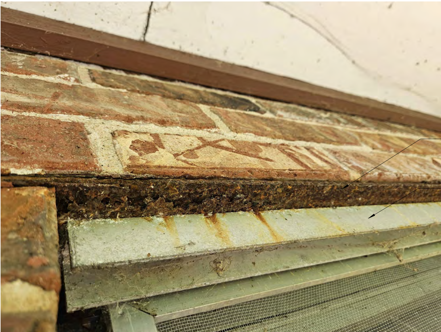
EXAMPLES OF RUSTED LINTELS: BUSSE FOREST WEST GROVE #31
