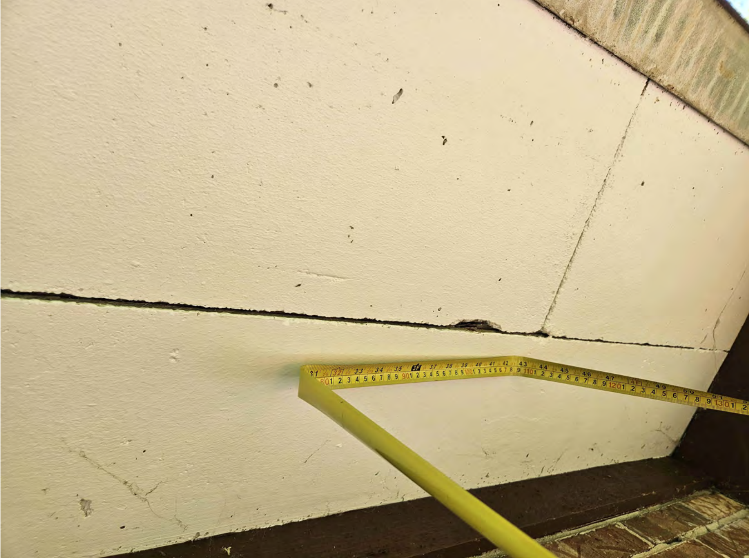
EXAMPLE OF PRECAST CONCRETE WITH GAPS BETWEEN PANELS TO BE RECAULKED: BUSSE FOREST WEST GROVE #31
