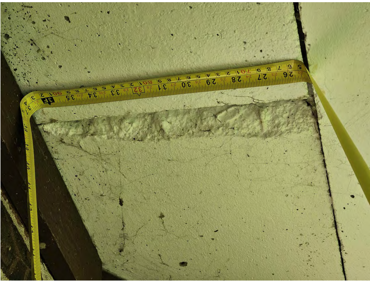
EXAMPLE OF PRECAST CONCRETE OVERHANG TO RECEIVE PATCH AND REPAIR - BUSSE FOREST SOUTH GROVE #4: EXTERIOR SOFFIT
