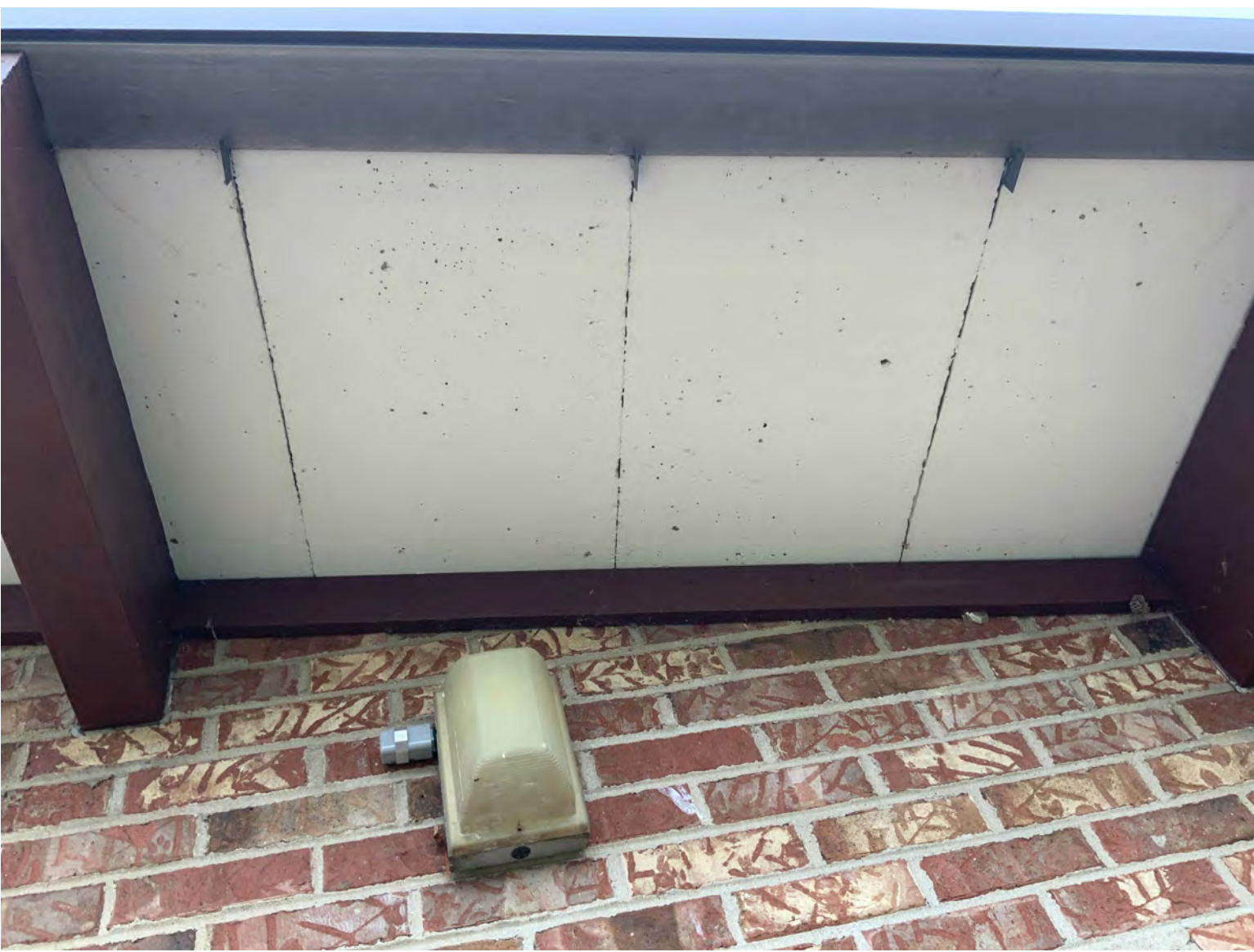
EXAMPLE OF PRECAST CONCRETE WITH SEAMS BETWEEN PANELS TO BE RECAULKED: BUSSE NED BROWN GROVE #28
