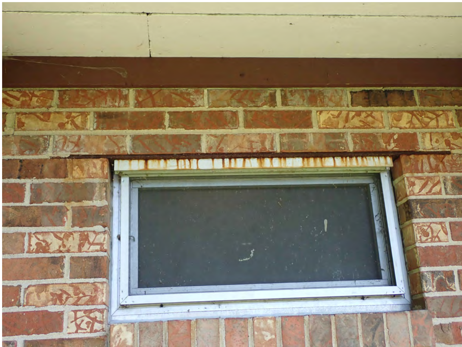
EXAMPLES OF RUSTED LINTELS TO BE CLEANED, SANDED, REFINISHED: BUSSE FOREST WEST GROVE #31
