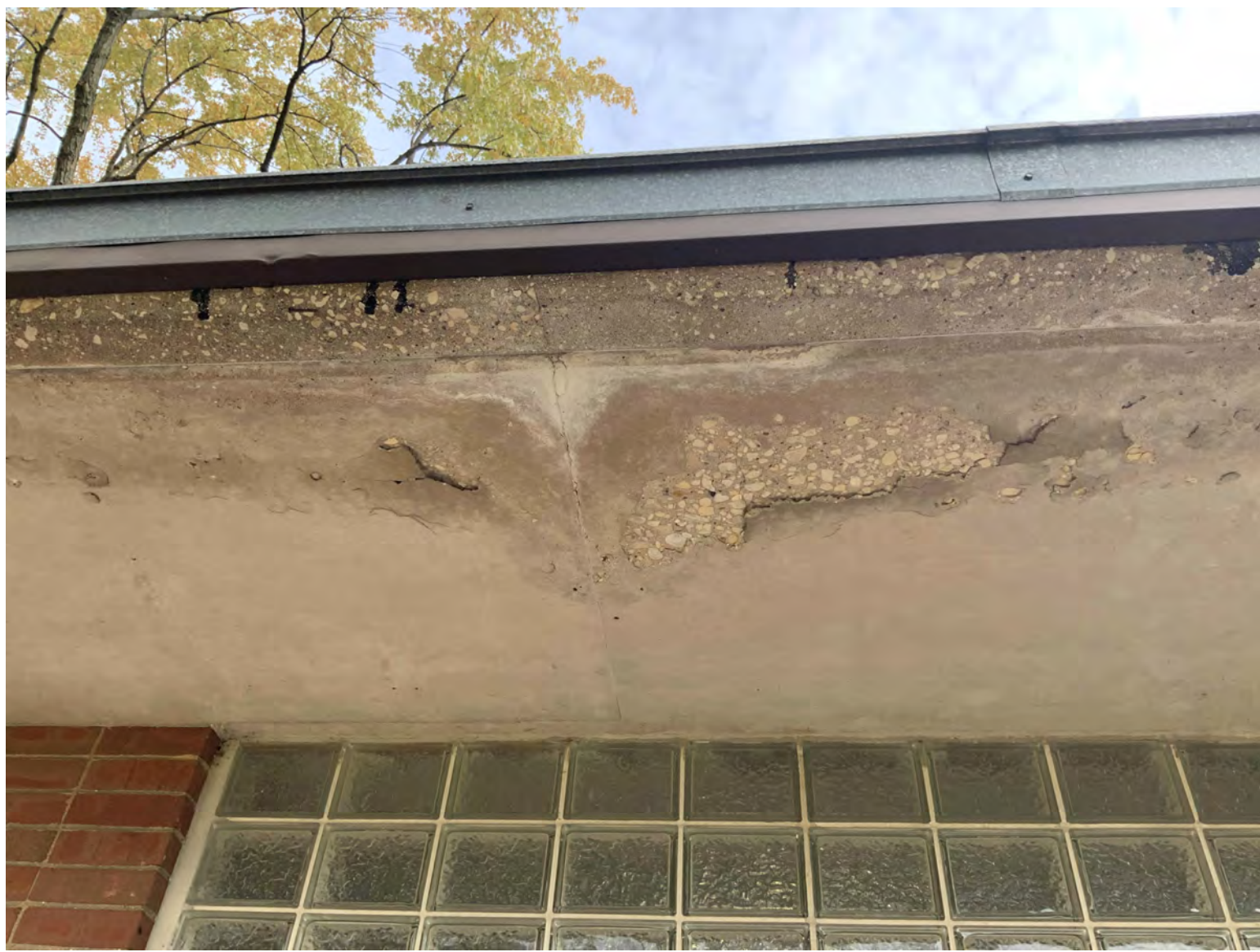
EXAMPLE OF DELAMINATING CONCRETE ON PRECAST OVERHANG, PROVIDE CEMENTITIOUS PATCHING AND REPAIR MATERIALS + REPAINT: DAN RYAN WOODS GROVE #2
