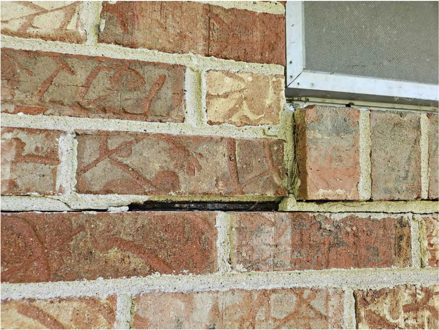
EXAMPLES LOOSE MORTAR TO BE REPLACED: BUSSE FOREST WEST GROVE #4
