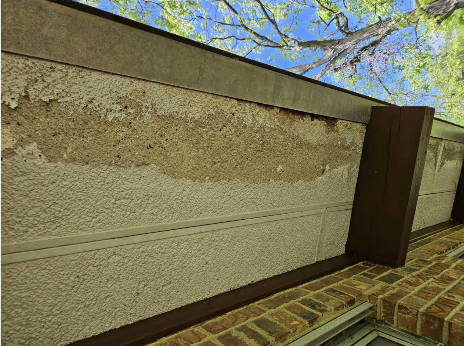
EXAMPLE OF PRECAST CONCRETE OVERHANG IN NEED OF PATCHING AND REPAINT - BUSSE FOREST SOUTH GROVE #24: EXTERIOR SOFFIT
